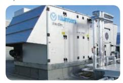
The FreeDry<sup>™</sup> system uses the condenser side of a heat pump circuit to reactivate a desiccant dehumidification wheel. The efficiency of this cycle provides an extremely efficient reactivation input.
