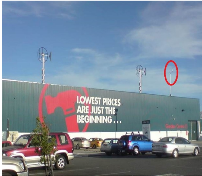
Figure 2a. A photograph of the front view of the Bunnings warehouse showing the five small wind turbines and the ultrasonic anemometer position (red circle).
