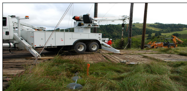
BPA installs temporary wood mats over wetlands to minimize impacts from heavy vehicles and equipment during construction of transmission line structures.
