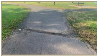
Figure 49. Cracked walking trail.
