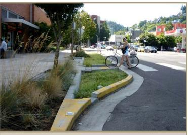
*Figure 17. Green infrastructure used to narrow the roadway and provide a shorter crossing distance for pedestrians.*
