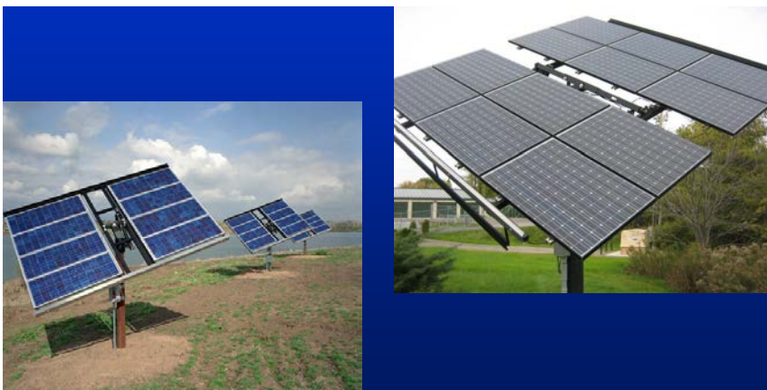
Figure 24. Sun-tracking arrays are typically mounted on poles and increase the amount of solar energy received.
