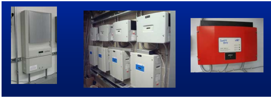
Figure 73B. String inverters are small inverters in the 1 to 12 kW size range, intended for residential and small commercial applications.
