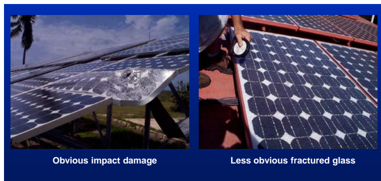
Figure 109. Inspect PV arrays for any signs of physical damage, such as impacts or fractures.
