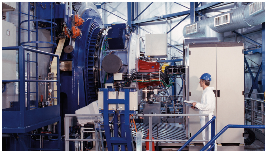
Figure 1. NAOS (light blue) and CONICA (red) are attached to the Nasmyth B adapter of UT4 (Yepun). The control electronics are housed in the white cabinets.
