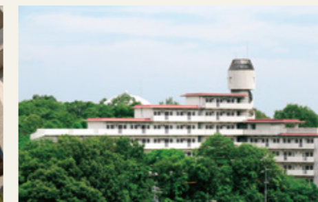
International Residence HIGASHIYAMA
