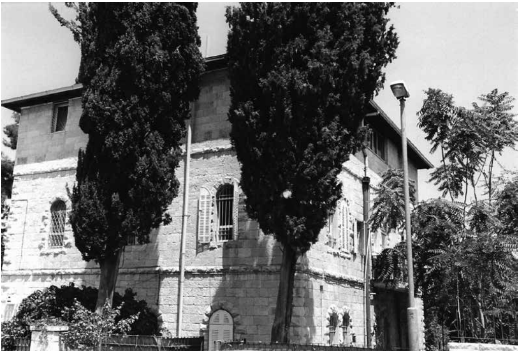
Figure 6. Cnaan’s house in al-Musrara. The third floor was added by the occupying Israelis after 1967. Located within the Armistice Zone in the No-Man’s Land just below the Notre Dame de France, the house was damaged and inhabited between 1948 and 1967. The street’s name during the British Mandate was Godfrey de Bouillon Street, while the present Israeli name is Ha’ Ayim Het Street. Photo taken in 1998, courtesy of Fauzi Mantoura.
