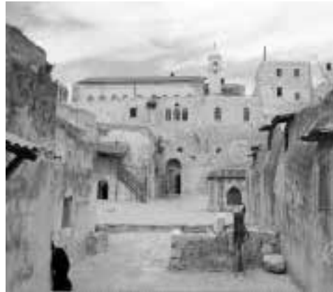
Figure 2. Ethiopian monks' rooms on the roof of the Holy Sepulcher.
