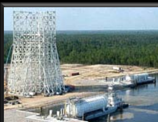
Test Stand A-3 structure
