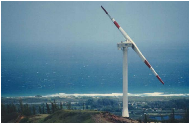
A two blade turbine specifically developed for hurricane-prone areas.
