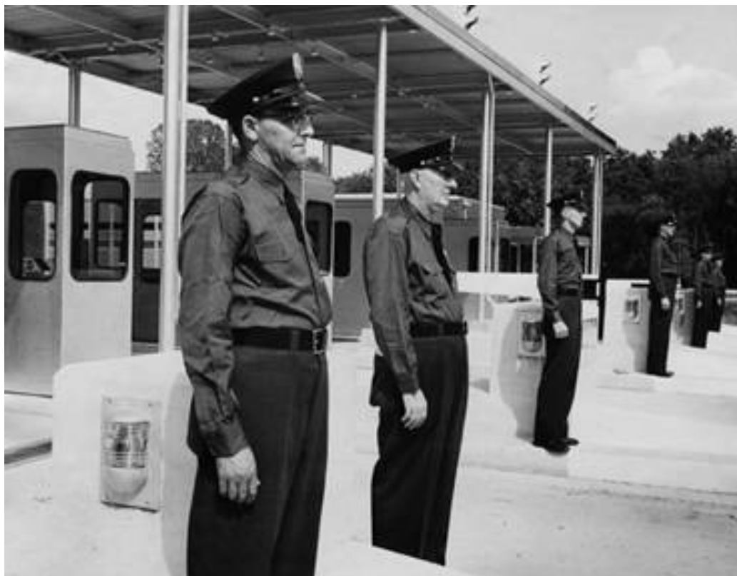
Figure 1. Toll booth operators ready for duty on the Richmond-Petersburg Turnpike, June 1958 ( Richmond Times-Dispatch ).
