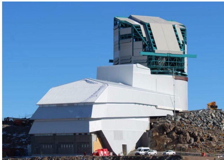
While the COVID-19 pandemic forced a suspension of summit construction activity of Vera C. Rubin Observatory, the project maintained regular inspections of the site. This photo was taken during the inspection conducted on June 9, 2020. Credit: Rubin Observatory/AURA/NSF.
