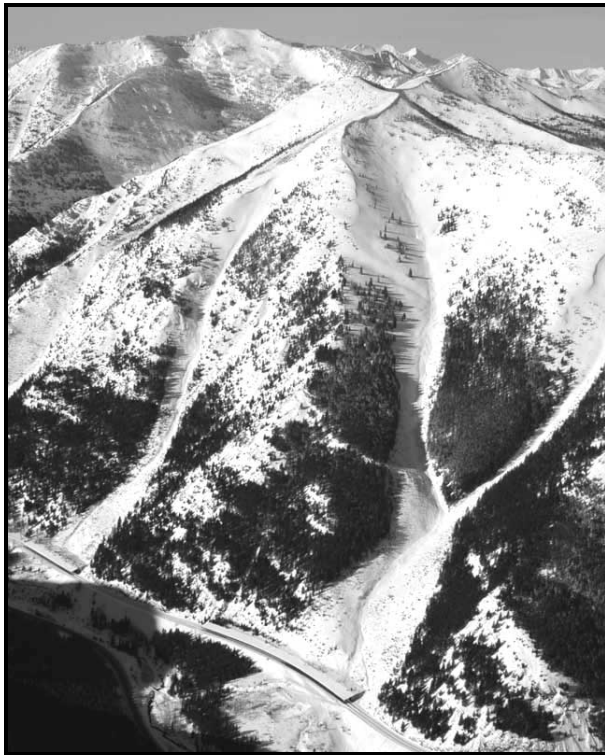
Figure 5: Aerial photo showing (L-R) Shed 8 and Shed 7 avalanche paths on Snowslip Mountain, with cornices formed by prevailing west winds. Visible in lower center is east end of Shed 7, where slides have blocked entrance to the shed numerous times. Photo by D. Stoneman.
