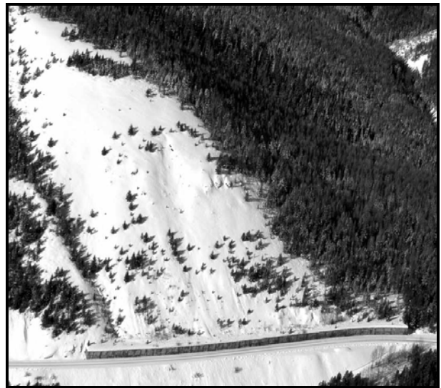
Figure 6: Aerial photo of burned-out snow shed (4-C) showing steep, unconfined avalanche path. Photo by D. Stoneman.
