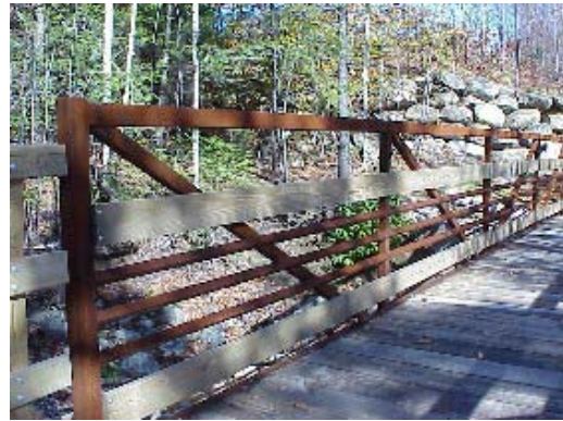
Figure 3: NH White Mountain Trail Bridge
