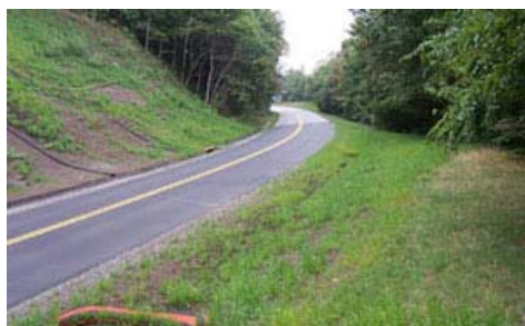
Figure 19: Compost Blanket on Steep Slope on Federal Highway Helped Restore Slide and Re-establish Vegetation Restoration Despite Severe Drought
