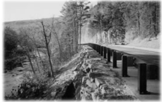
Figure 4: Arkansas SHDT Historic Bridge and Native Stone Retaining Wall
