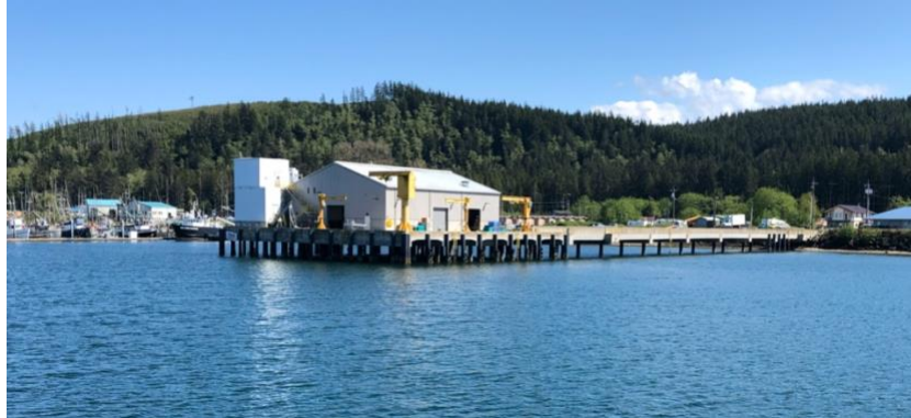
Figure 2. Dock constructed in Phase 1 of the project (Source: Makah Tribe, 2020)
