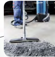
Dust extraction and cleaning
