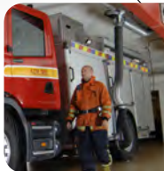
Vehicle exhaust extraction
