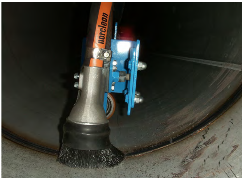
Fig. 3. The on-tool vacuum blaster is suitable for blasting welding-joints.
