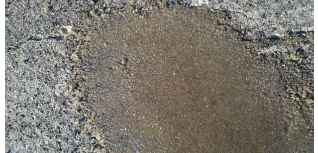
Patched with Epoxy & Sand
