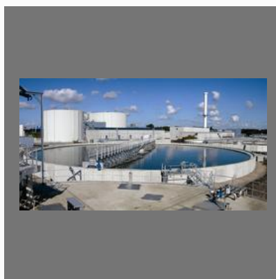
Industrial Waste Water Treatment Plant
