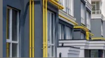
Natural Gas Pipeline Installation Service
