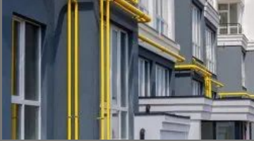
LPG Gas Pipeline Installation Services
