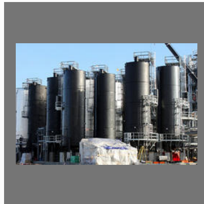
Carbon Steel Tank
