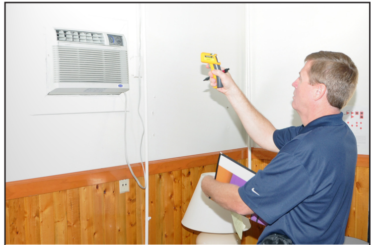
Tom Riney, senior energy engineer, SAIN Engineering measures discharge and return of air from an air conditioning unit while collecting room temperature using an infrared thermometer
