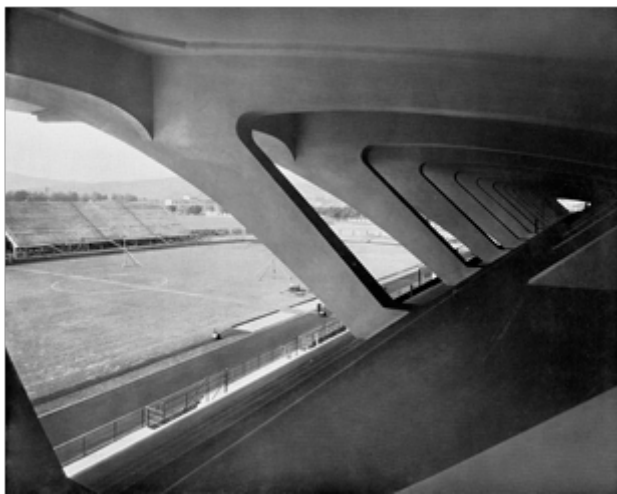
Figure 6. Interior view showing the bifurcating beam and its connection to the longitudinal stiffening beam. (book Structures , New York: Mc-Graw Hill, 1955.)
