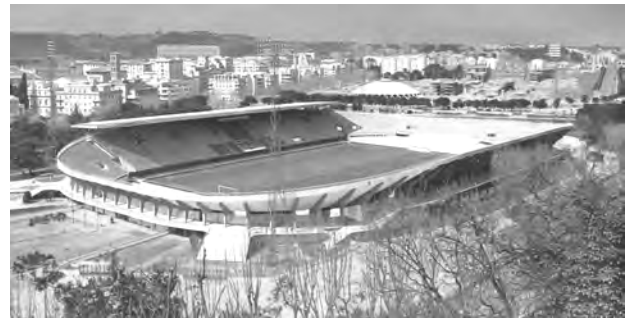
Figure 8. An overall view of the Flaminio stadium shows the standing grandstands on the short side of the ellipsoid floor plan and the covered grandstand on one side. (book New Structures, London: Architectural Press, 1963)
