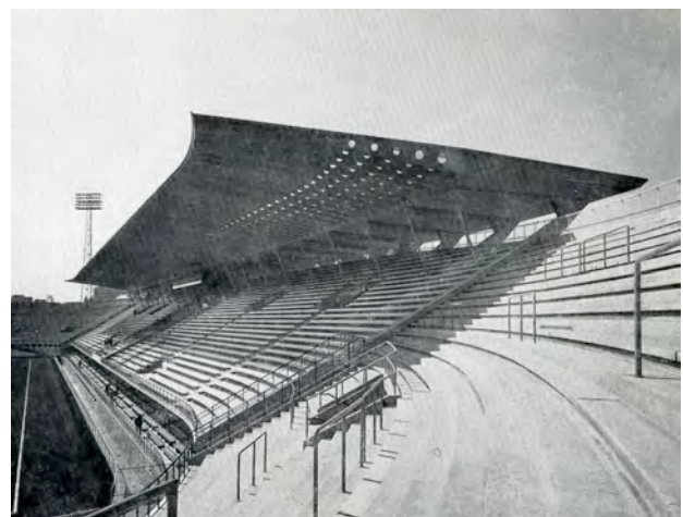
Figure 9. Perspective of the cantilevering roof showing the web apertures in the ferro-cement beam and the interior steel column positioned far back. (book Ingg. Nervi & Bartoli, societa per azioni)
