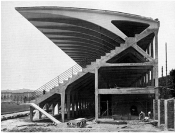
Figure 4. The stadium under construction shows the bifurcating cantilevering roof and the support frame. (book Ingg. Nervi & Bartoli, societa per azioni )
