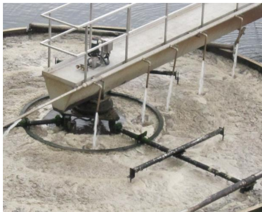
Figure 6 - Foam was fluidized with sprays and forced below the surface.
