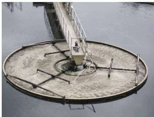
Figure 5 - Suspended solids and foam were accumulated and floated inside the energy dissipating inlets and flocculation centre well respectively.
