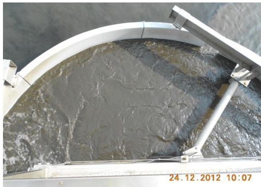
Figure 14 - No foam was observed at the final clarifier with new FCW design (24 December 2012).
