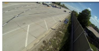
South DLT (West) Side – Looking Southeast – CAM 13 – Start at 15:00:00 – Duration of 0:17:04
