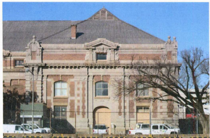
MAIN SEWERAGE PUMPING STATION
