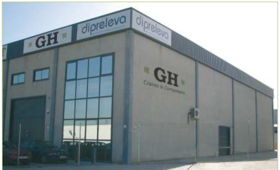
GH spare parts distribution center
