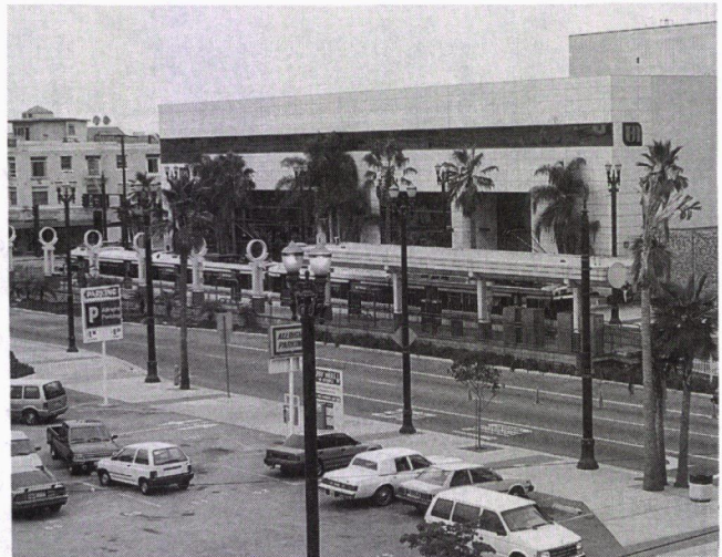
FIGURE 7 High-level platforms provide level entry to high-floor cars. Integrating such platforms into the city scene can be done attractively, as in Long Beach, California.
