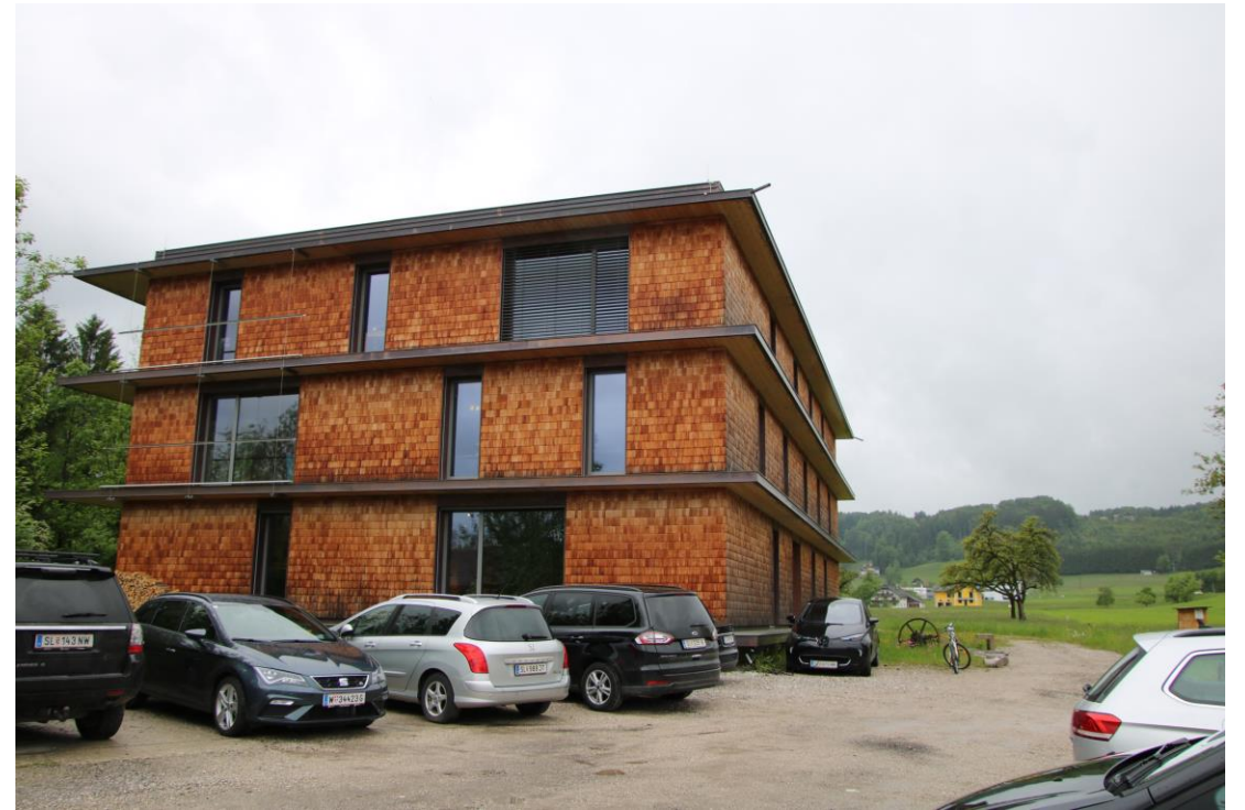
CLT structure in Austria
