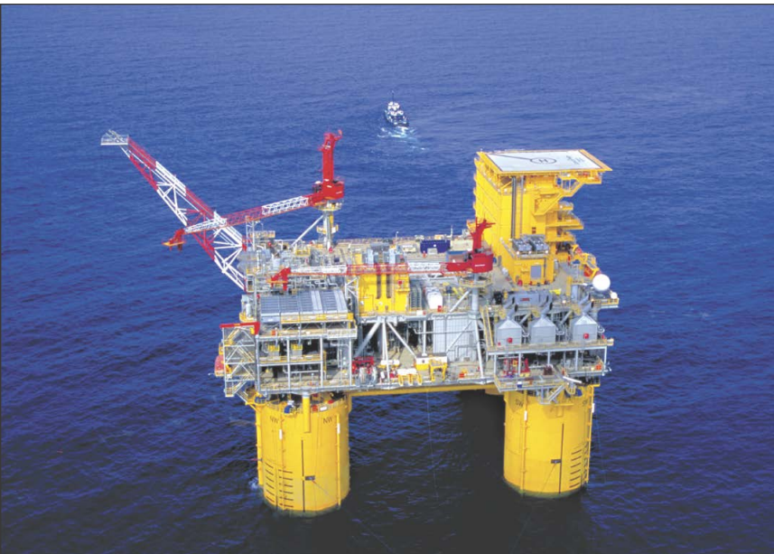
Replacing standard three-coat systems with two-coat systems in aggressive environments has been done occasionally, but such a move must be taken with great care.
