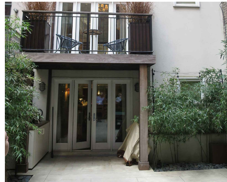
EXISTING REAR FACADE
