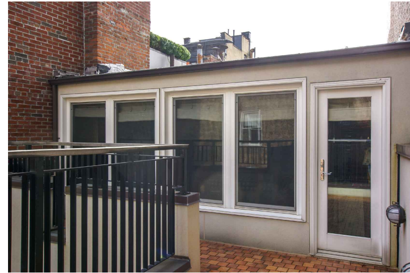
EXISTING REAR FACADE AT 5TH FLOOR
