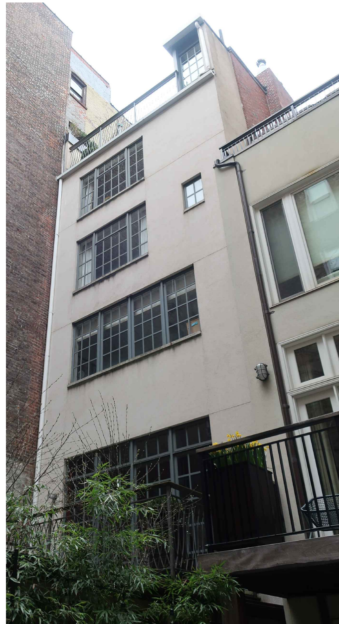
REAR FACADE AT 55 BANK ST
