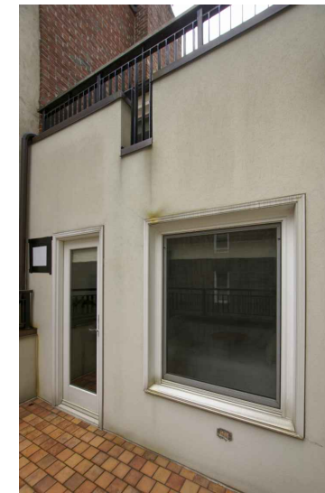
EXISTING REAR FACADE AT 4TH FLOOR
