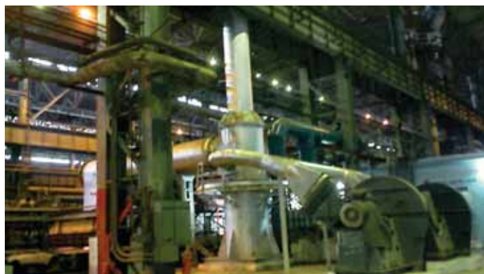
Fig 4 Furnace flue outlet and dilution air blowers connected to chimney
