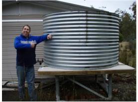
The inlet was attached to the top of the tank with a saddle to replace the ingeniously constructed pile of bricks and scraps of wood used before.
