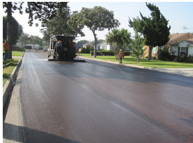
Slurry seal operation
