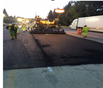
Night paving on I-5
