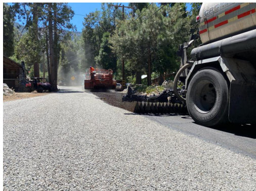
Chip seal operation
