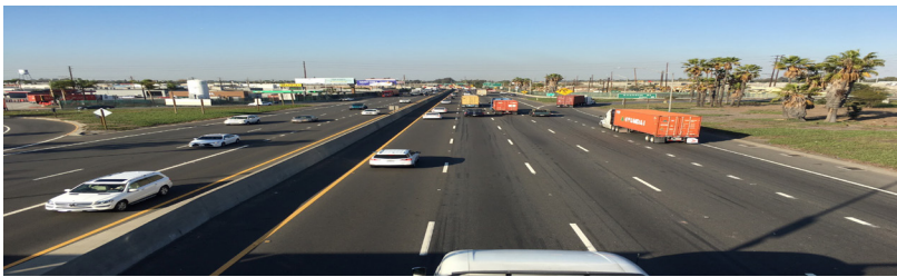
I-710 Long-Life Project after over 20 years of service
