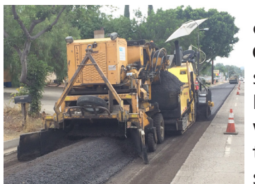
Figure 2. Windrow Paving of CIR Mix
