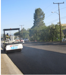
Thin Asphalt Overlay
