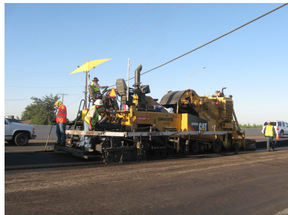
Thin Hot mix asphalt overlay
