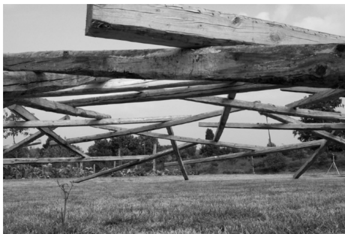
Fig. 5. Second dome completed
