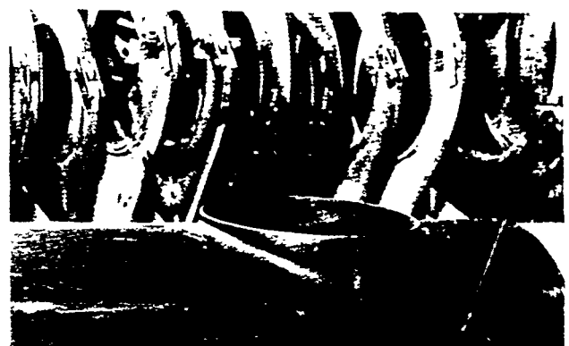
14 The collar is ready for butt welding.
