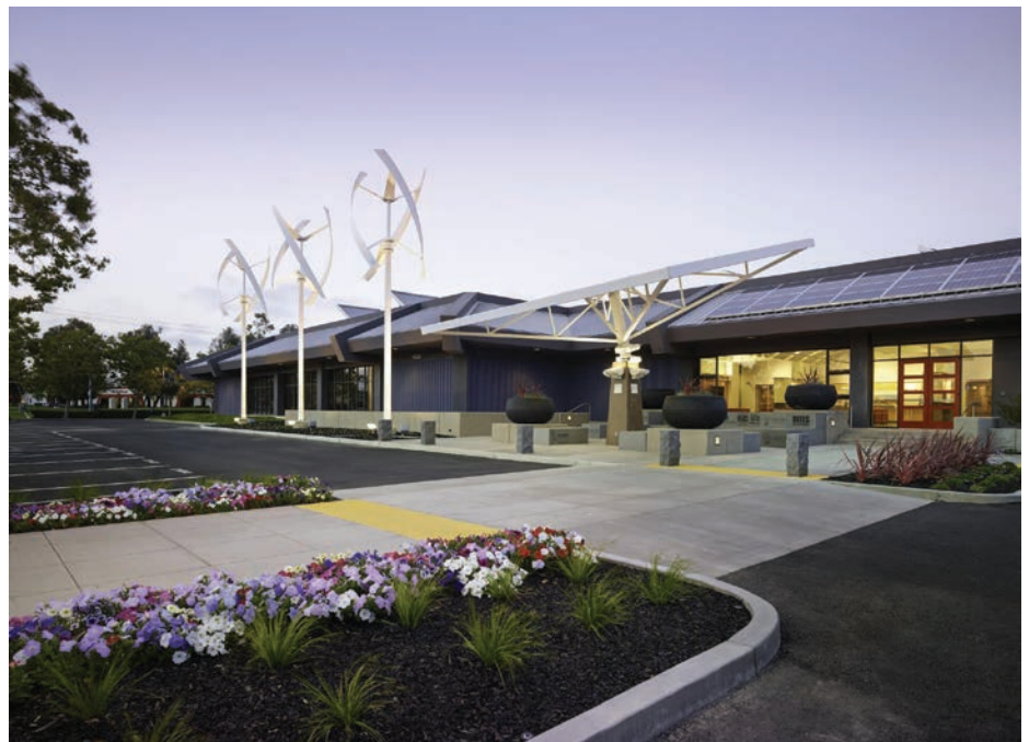
The Zero Net Energy Center leads the nation's sustainable building standards by planning to meet the California Energy Commission's 2030 Net Zero Energy Challenge 17 years ahead of schedule.
