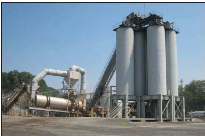
A modern hot mix asphalt facility provides high production, good quality mixes (including recycled asphalt pavement if desired) while meeting stringent air quality standards.
