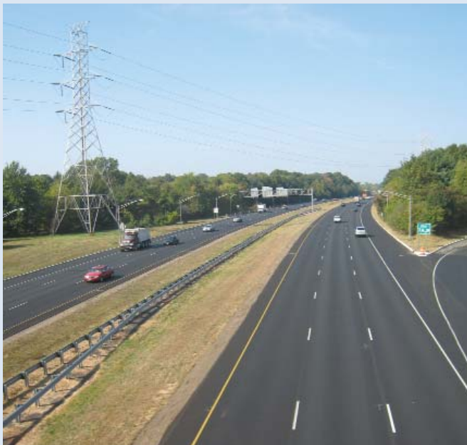
NJDEP Award Winning Asphalt Rubber Mix Used on Route 95 in Central New Jersey
