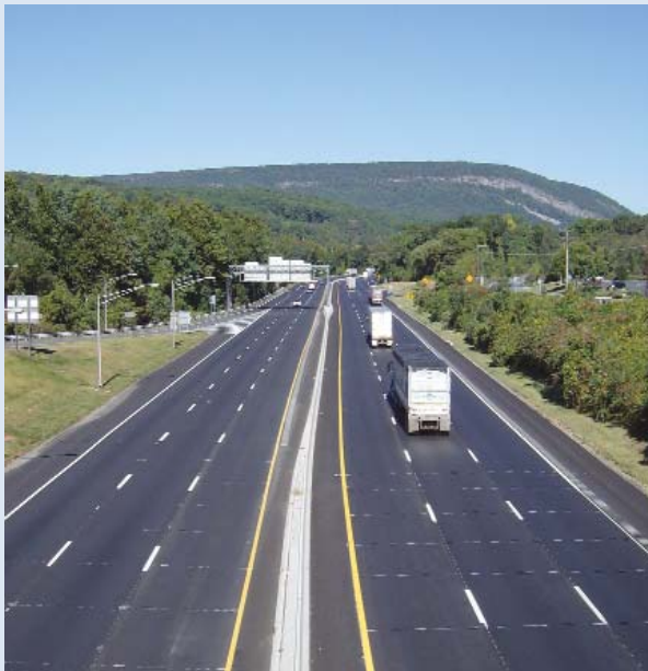
Stone Matrix Asphalt application on Route 80 in Northern New Jersey
