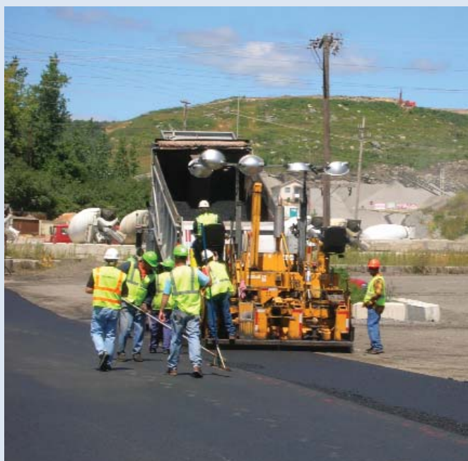
Warm Mix Asphalt application used in Northern New Jersey
