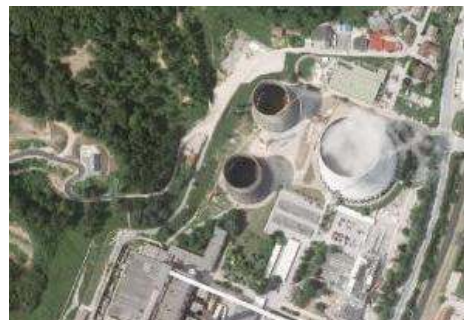
Satellite picture of TES area, Photo taken from Google Maps, 2012
