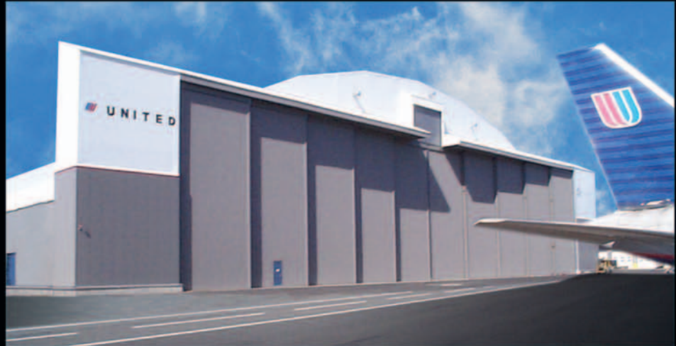
240' W x 55' H, 10-leaf, bi-parting Door System with tail door
