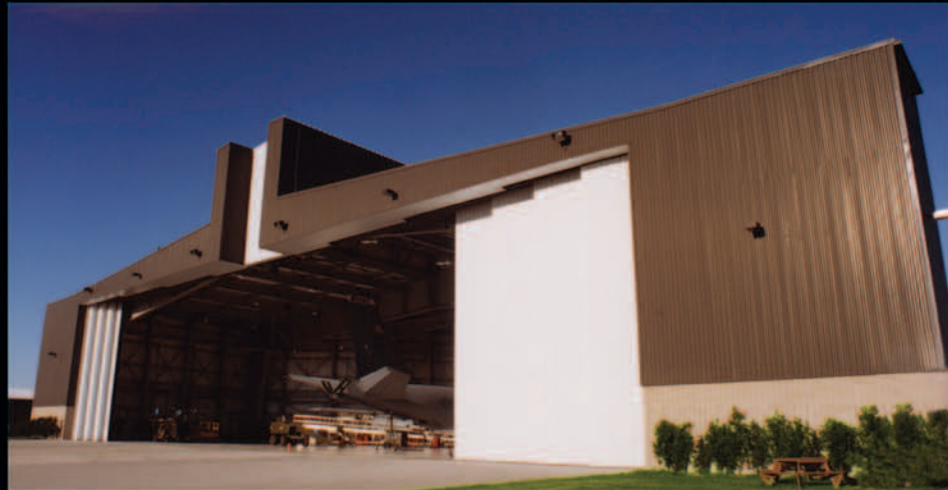
195' W x 43' H, 8-leaf, bi-parting Door System with tail door
