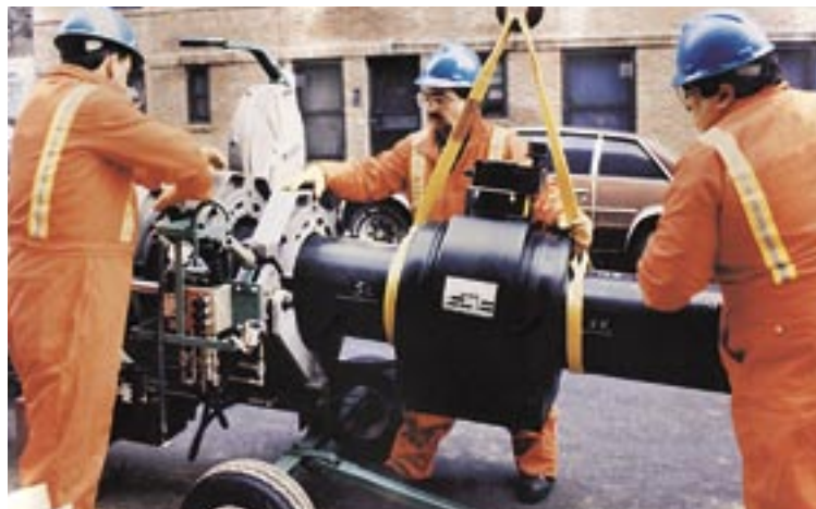
12" Poly-Gas ® valve installation
