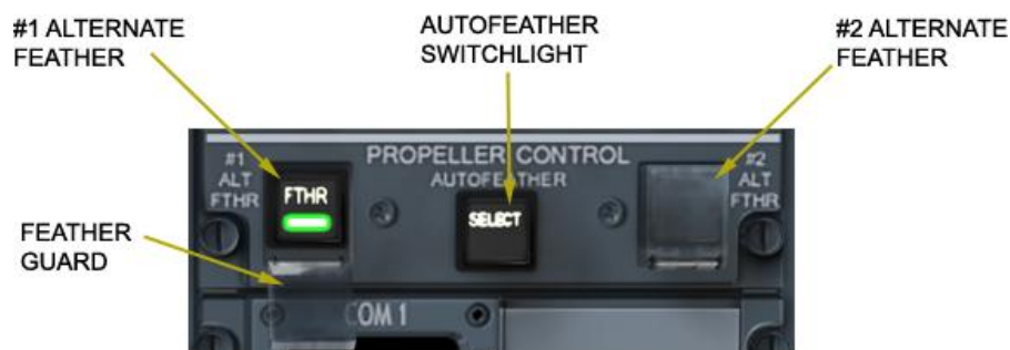
Figure 15.3.4.1. The Propeller Control Panel
