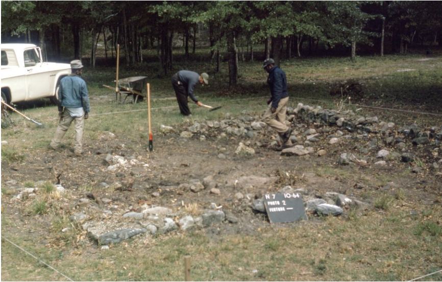
Figure 4. Beginning the excavations on the Courthouse ruin at Brunswick Town in 1964. View faces west.
