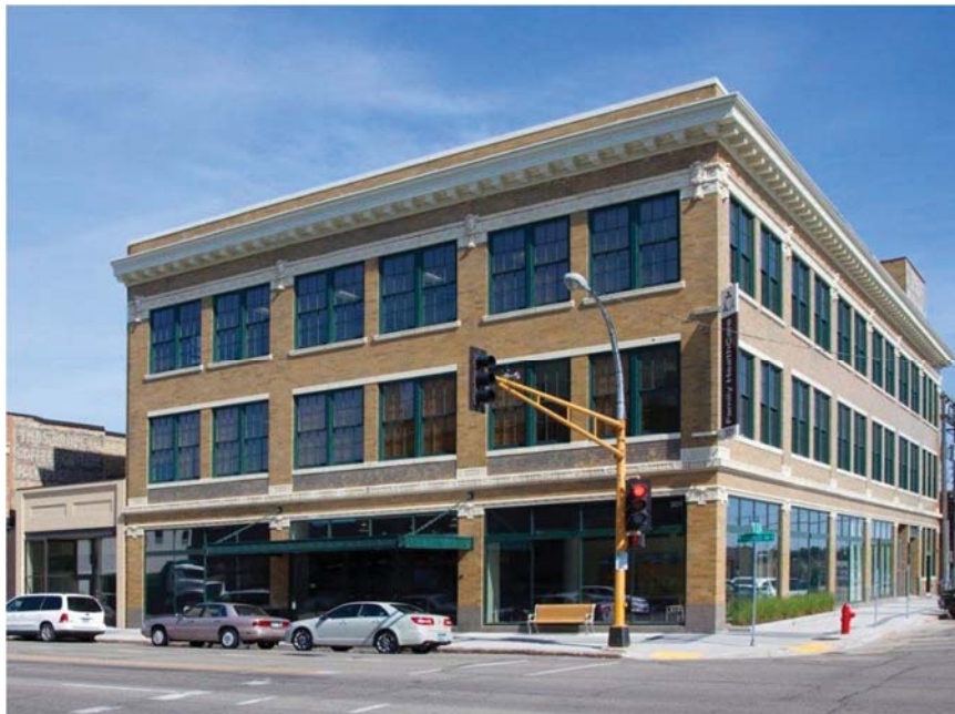
Pence Automobile Building, 310 NP Avenue, Fargo, North Dakota (rehabilitated for use as a healthcare facility in 2011 by the Kilborne Group)
