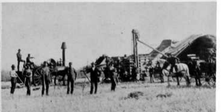
Swinging Straw Stacker, used before the blower was invented.
