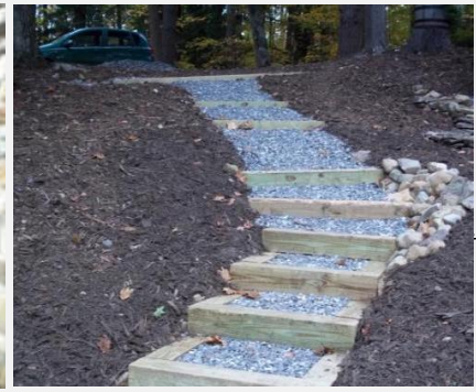
Infiltration Steps Protect Steep Slopes w/Foot Traffic
