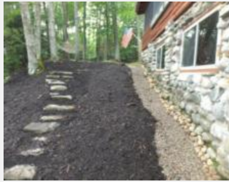
Dripline Trench & Erosion Control Mulch
