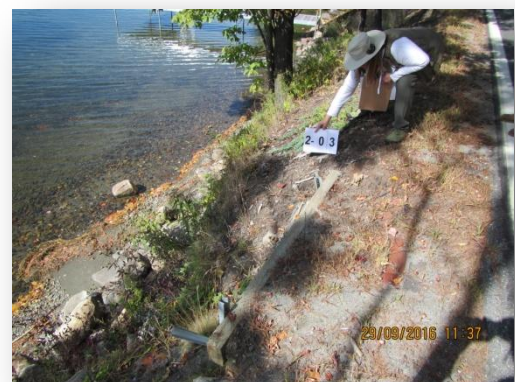
Example of a narrow stretch of land between the state road and the lake used for beach/boat access.
