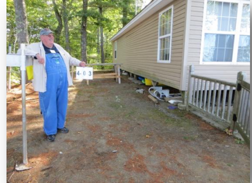
Bare soil & roof runoff in Sector 4.
