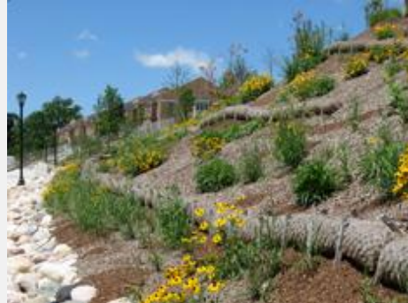
Erosion control blankets, coir logs & vegetation to stabilize slopes
