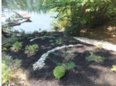
Erosion Control Mulch & Vegetative Plantings
