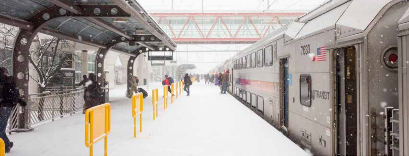
NJ TRANSIT's Hamilton Station in New Jersey
