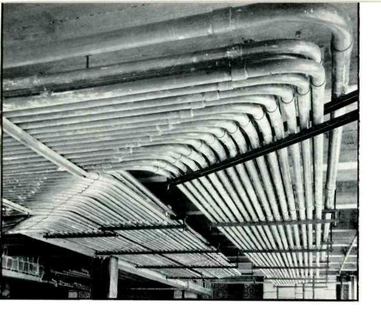
Pipes for television: Above, 80 2-inch and 3-inch conduits installed at Radio City in 1933 for future television facilities. Below, coaxial line cords, jacks, and plugs, showing the termination of the Fifth avenue coaxial cable (main equipment room)
