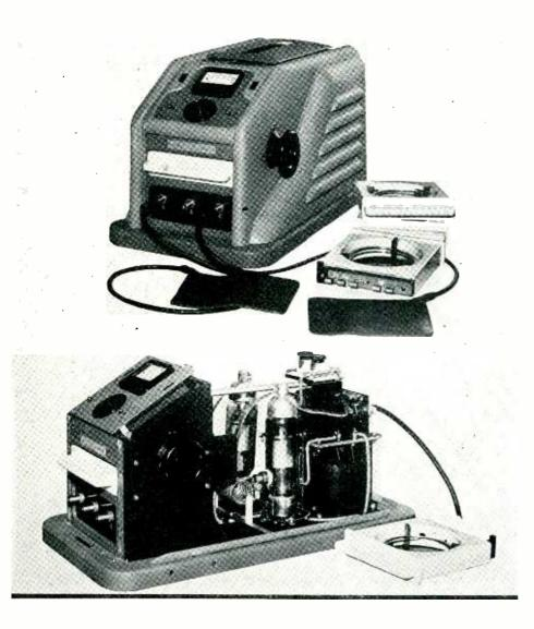
Above: The interchangeable coils permit operation between 5 and 18 meters. The knob on the side of the unit controls output which is measured by the meter. The control just below the meter is a time switch which automatically determines length of treatment. Below: Interior view of half-kilowatt diathermy machine. The power supply is at the right. A portion of the oscillating circuit can be seen to the left of the tubes
