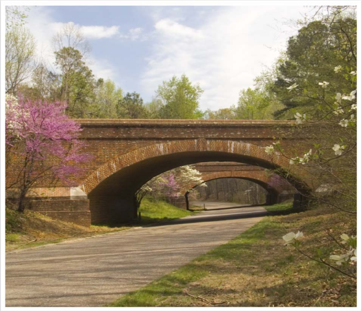
View of Colonial Parkway Bridges at the Colonial National Historic Park, Virginia credit: NPS photo
