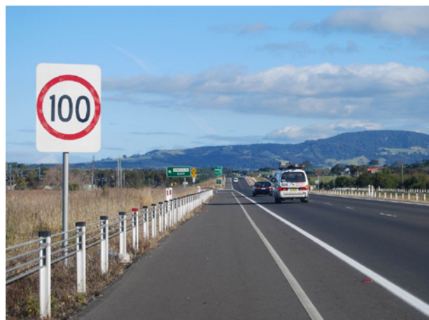
FIGURE 3.9 RURAL DIVIDED ROAD
