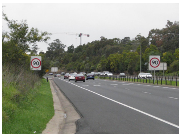
FIGURE 3.8 HIGH VOLUME URBAN MOTORWAY
