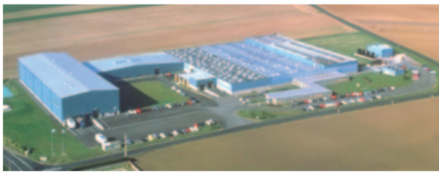
Camfil Farr production plant Saint-Martin Longueau, France
