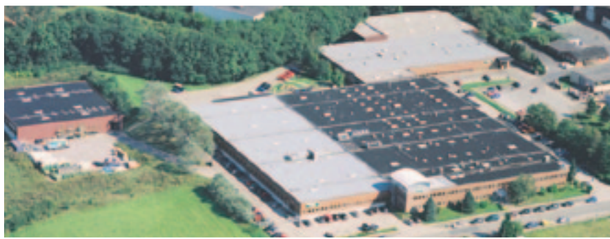
Camfil Farr production plant Reinfeld, Germany
