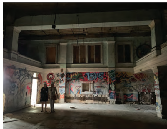
View of the south courtroom. The courthouse features three, all of which must generally be retained in their historic configurations.
