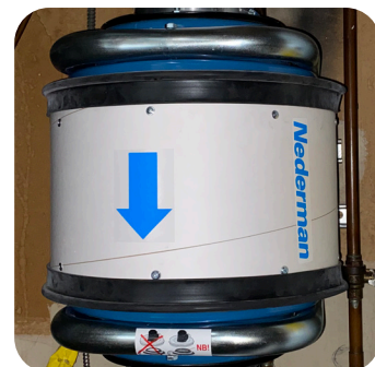
Nederman FX 2 HEPA filter is installed away from the patient area in the mechanical room.
